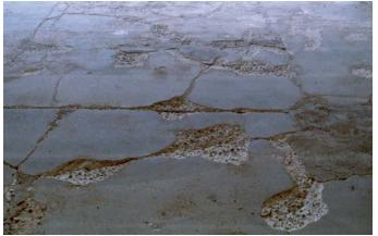
Recodi offers the best solutions for the maintenance and repair of damaged and obsolete surfaces. Thanks to advanced technologies, we are able to breathe new life into your floors 3. Breakage and detachment of industrial tiles (porcelain stoneware, clinker bricks, tiles)
