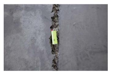
2. Low wear resistance with degraded surfaces, formation of holes and production of dust
